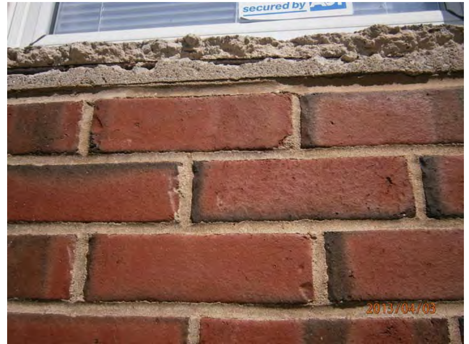
2. Damaged stone sill - exposed rebar
